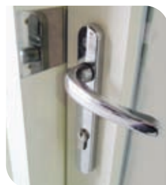
Locking handle and door striker plate detail
