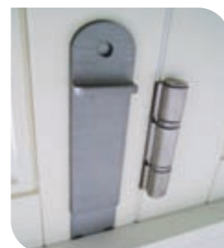
Dropbolts and internal hinge details
